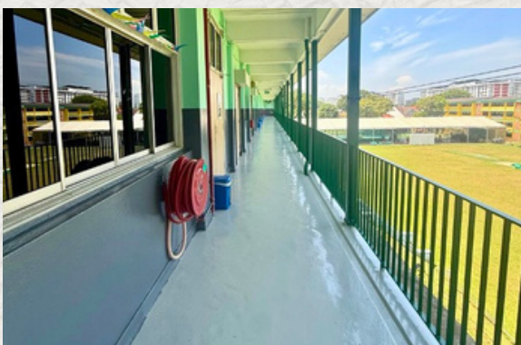
The long, bright, corridor open to the outside.
